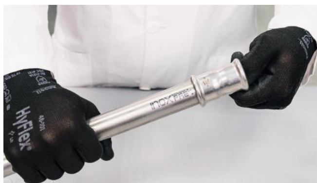
Figure 31 - Inserting pipe into the press fitting
