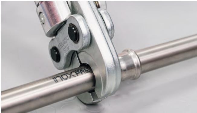
Figure 32 - Making the press connection
