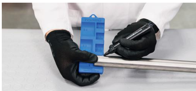
Figure 28 - Marking the insertion depth
