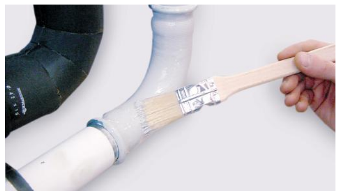
Figure 37 – Varnish of the connections and pipes with primer.
